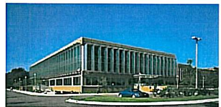
Walgreens corporate headquarters campus in Deerfield Illinois..
